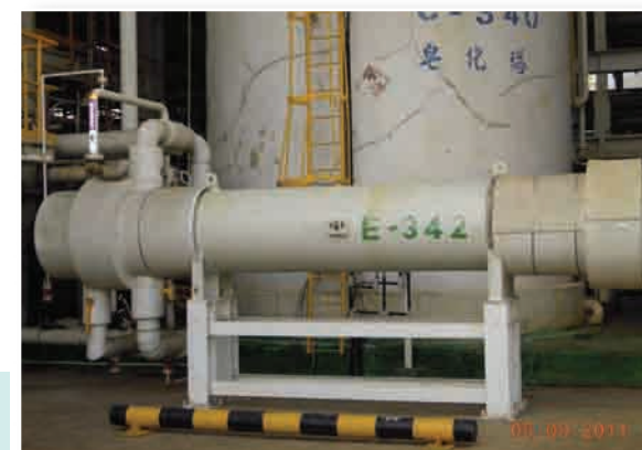
皂化塔液鹼入料預熱節汽改善
