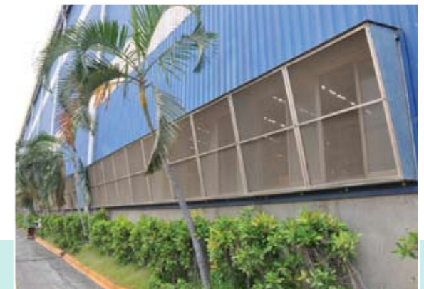
廠房通風節能之防塵防雨設計進氣窗
